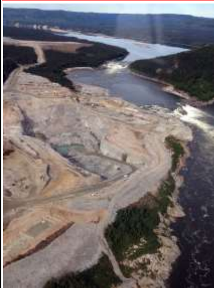
The excavated site at Muskrat Falls
